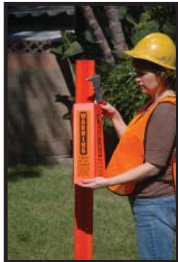
Fold panel into triangular shape and attach to the installed marker.
